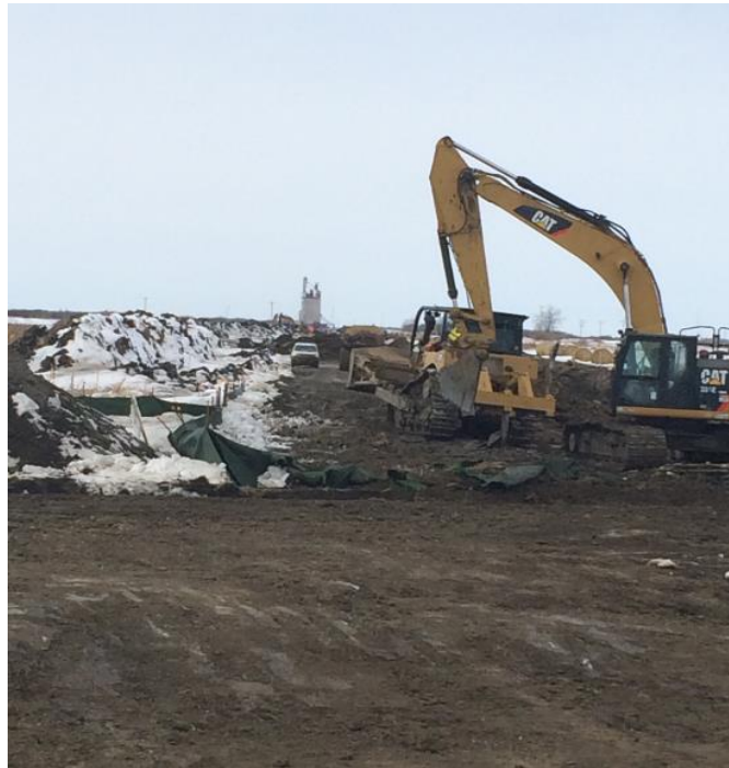
772 + 700 SK 908 Class IV Ramp removed
