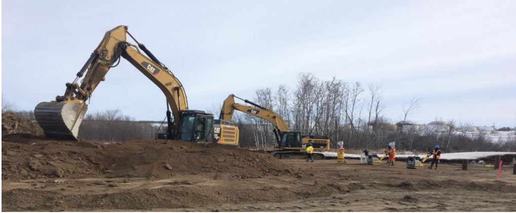
805 + 300 MLBV #23A Backfilled and packing.
