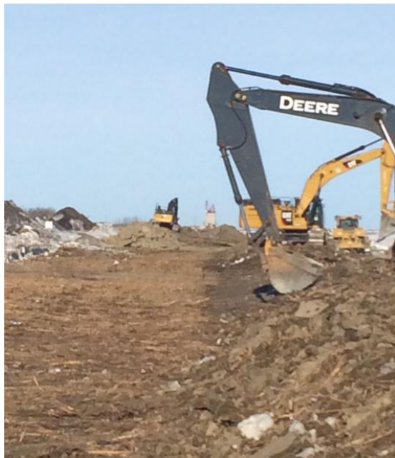
775 + 150 SK 911 Class IV Ramp removed
